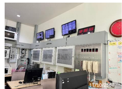
Graphic Annunciator Fire Alarm System
