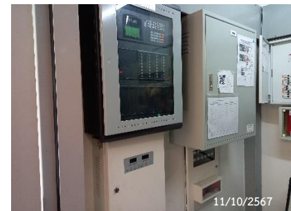
Fire Alarm Control Panel
